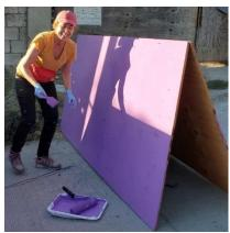
There are also four sheets of shorter plywood (4'x 75") for interior walls, these can be painted on both sides with the INTERIOR paint.
